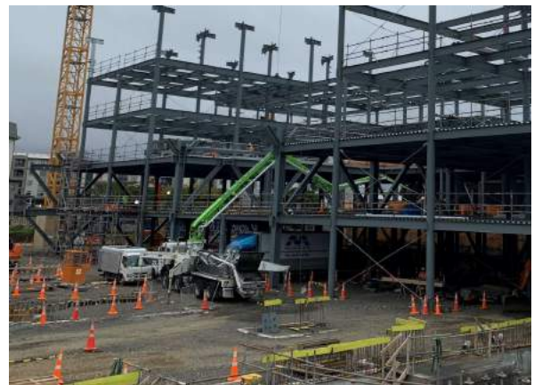
Concrete truck pouring the level 1 floor.
