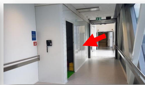
Hoarding on ESC sky bridge
