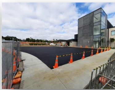
ESC temporary loading dock
