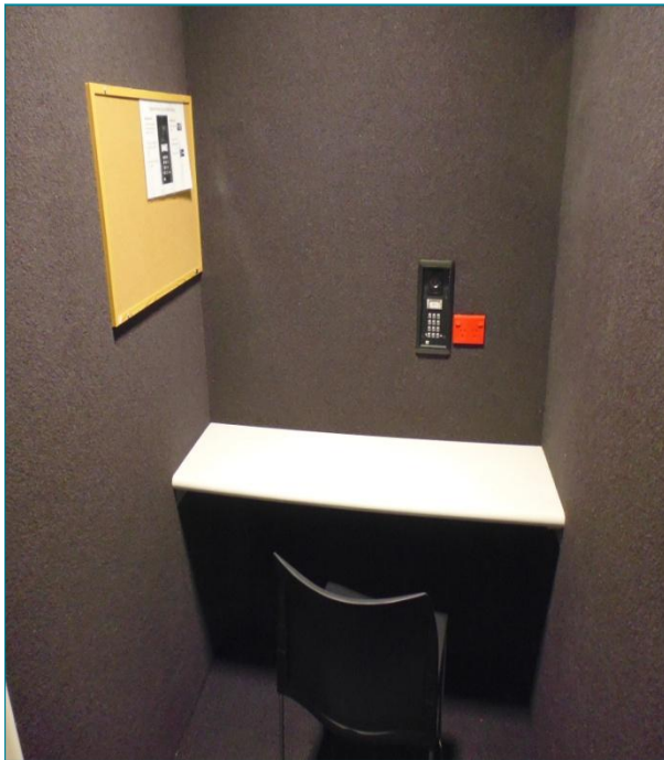
Figure 13: Telephone booth – not working
