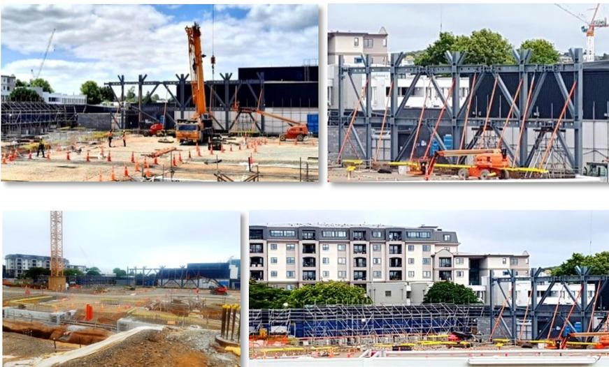
*Seismic k-bracing structural steel being installed on-site*
